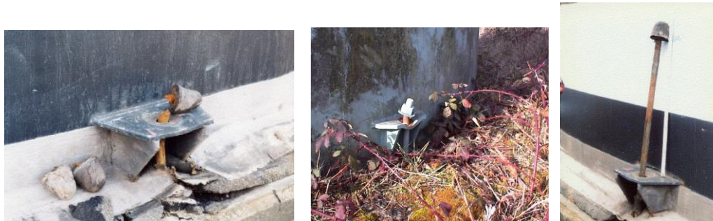
Figure 14: Anchor bolt failure in seismically-loaded tanks.
