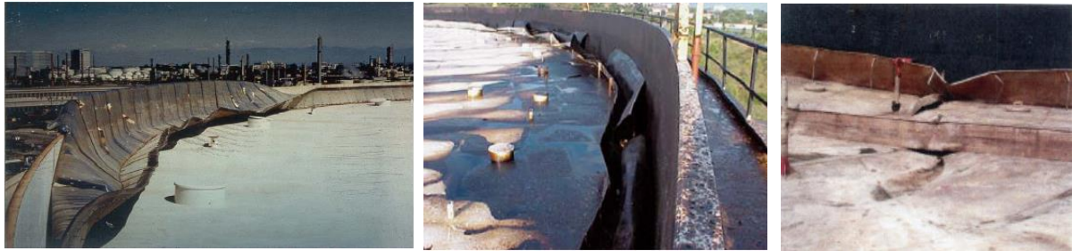
Figure 16: Failure of floating roof.
