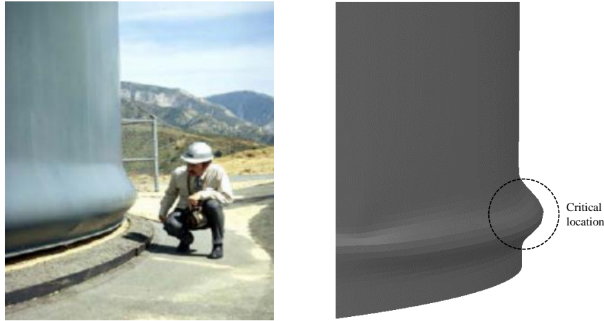
Figure 17: Elephant's foot buckling in liquid storage tanks (a) existing tank (Malhotra 2000), (b) buckling shape from present finite element analysis.
